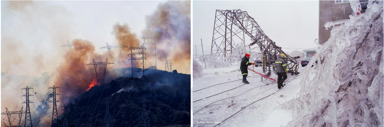
Figure 6: Experiences from forest fires [19] to ice-storms [20] have shown how vulnerable electricity grids can be to extreme weather events. Building and community scale electricity generation and storage will be essential for making communities resilient to the shocks of extreme climate events.
