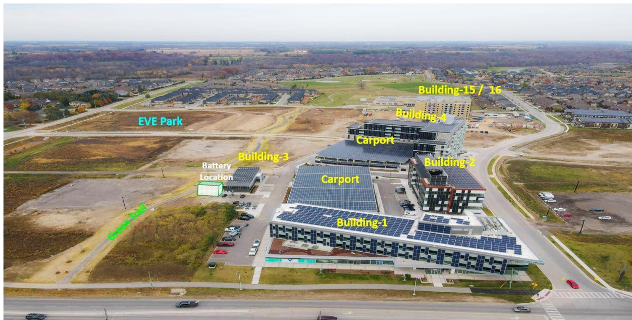
Figure 8: The partly completed West 5 development will be the first net-zero mixed-use community in Ontario.
