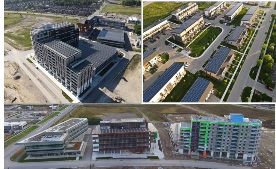
Pictures from West 5 (partly completed)
