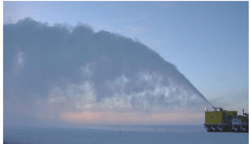
Ice Island Construction
