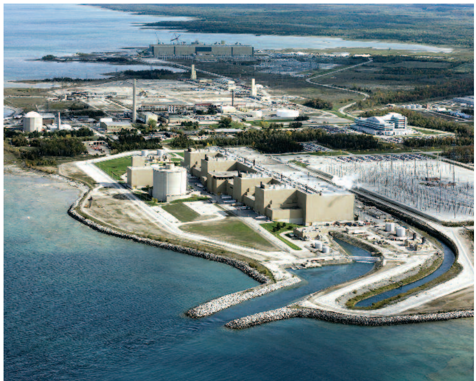
Figure 1 The Bruce Nuclear Power Development Site on Lake Huron
