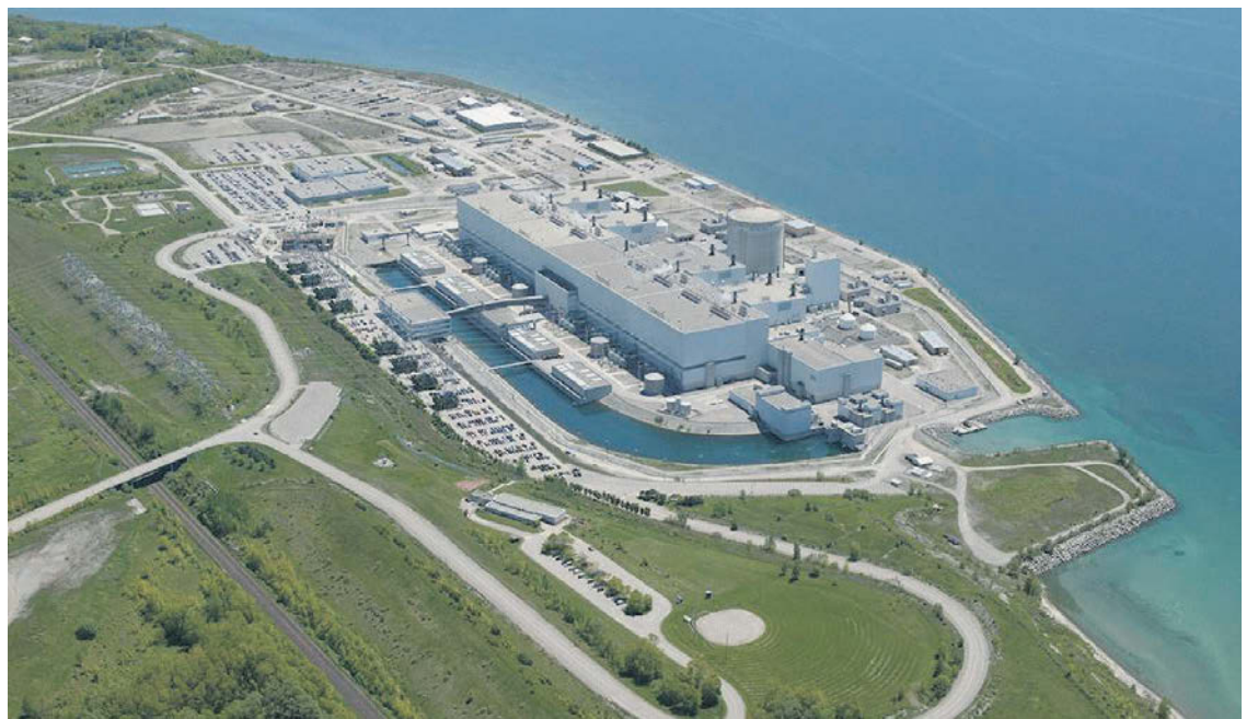
Located in the municipality of Clarington in Durham Region, 70 kilometres east of Toronto, Darlington is Ontario Power Generation's newest CANDU nuclear generating station. It provides approximately 20 per cent of Ontario's electricity needs, enough to serve a city of two million people. SUPPLIED
