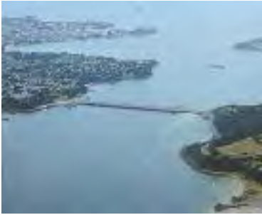
La Rance Tidal Power Plant in France
