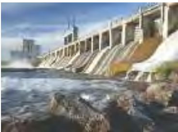
Seven Sisters Generating Station, Manitoba
