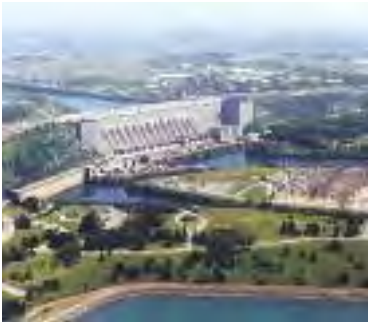
Sir Adam Beck Hydroelectric Project
